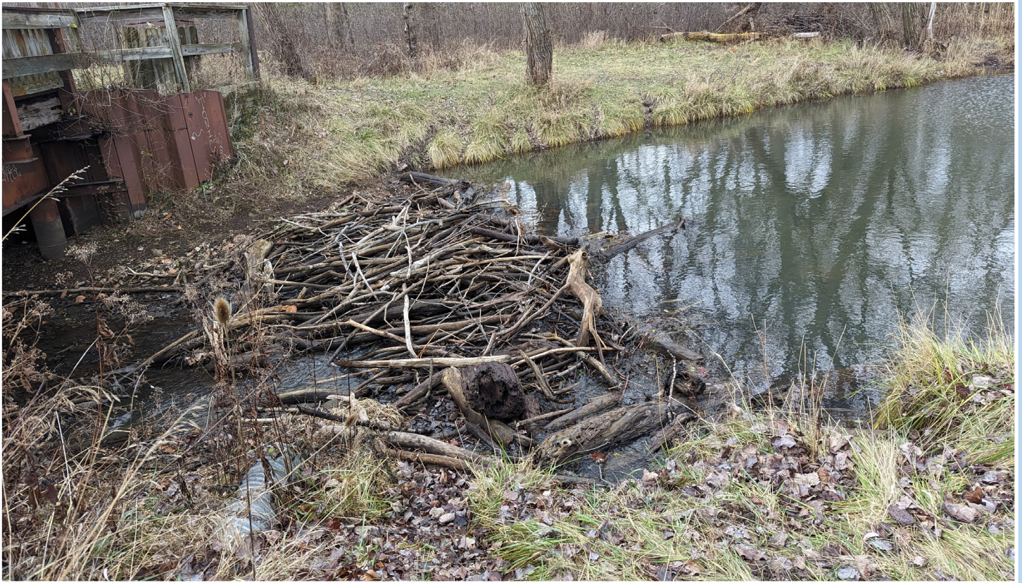
Figure 3: An abandoned beaver dam (estimated to be 2-3 years old) on a small creek. Beaver dams gradually deteriorate and become a part of the landscape. Ghost dams however, can obstruct streams over a hundred years after their original construction and need human intervention to be completely removed from the landscape. Photo: Roy Widrig.
