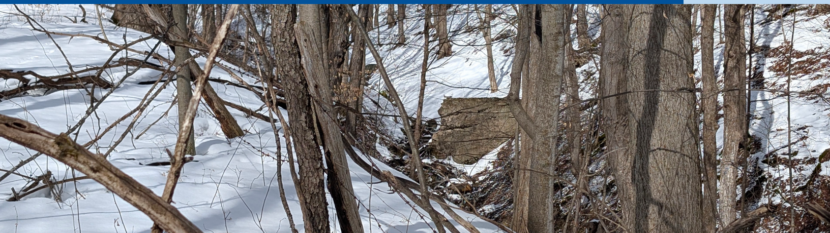
Figure 1: A ghost dam in a ravine, Central New York. This dam at an old summer camp no longer serves a purpose, but manages to retain sediment behind the remaining standing wall. Photo: Roy Widrig.
