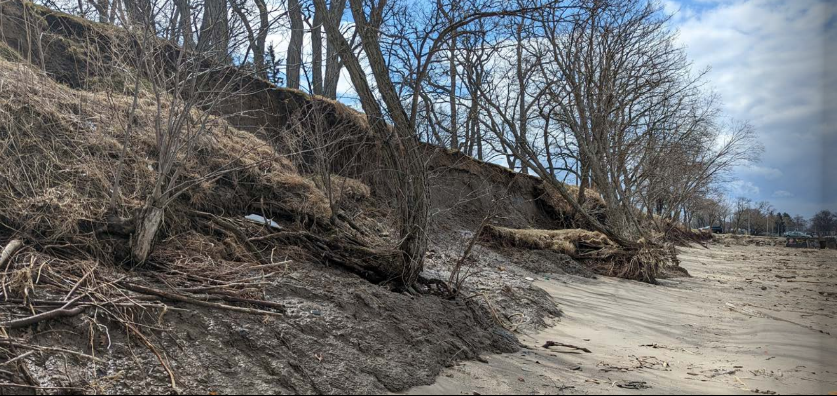
Figure 2. Oversaturated soils from intense rainfall or overwatering of lawns can cause soil to move away from and off of steep bluff faces in mass movements, sometimes as soil creep or earthflow (as seen above) but other times in small to large landslides (see insert.)
